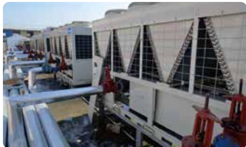
Grand Comfort Material Market Country: Kyrgyzstan Outdoor Units: Air-cooled modular chiller Indoor Units: FCU & AHU Total Capacity: 5,780kW Completion Year: 2015
